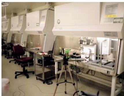
Figure 1. Newly installed Class II type A2 canopy-connected biological safety cabinets with HEPA-filtered supply air in close
